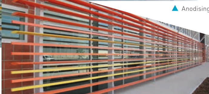
◀ Powder coated aluminium louvres supplied and installed for Brisbane City Council Bus Depot
