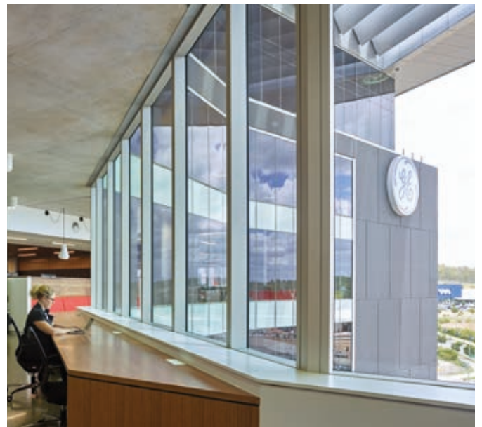
▲ Internal view GE Headquarters Springfield. GJ Solarplus (Low E on Grey) TwinGlaze units
