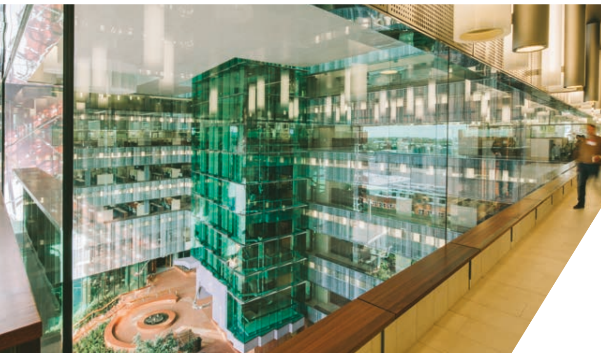
◀ Foreground: 586 Series custom designed 'Strongback' (mullionless) window system; Stairwell: Heat strengthened green laminate; All glazing by G.James Commercial Glass & Glazing; Translational Research Institute (TRI), Brisbane
