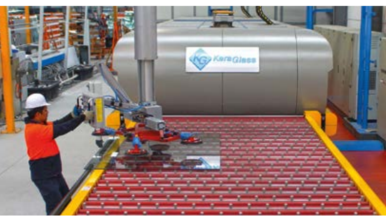
◀ Toughening furnace, Smithfield
