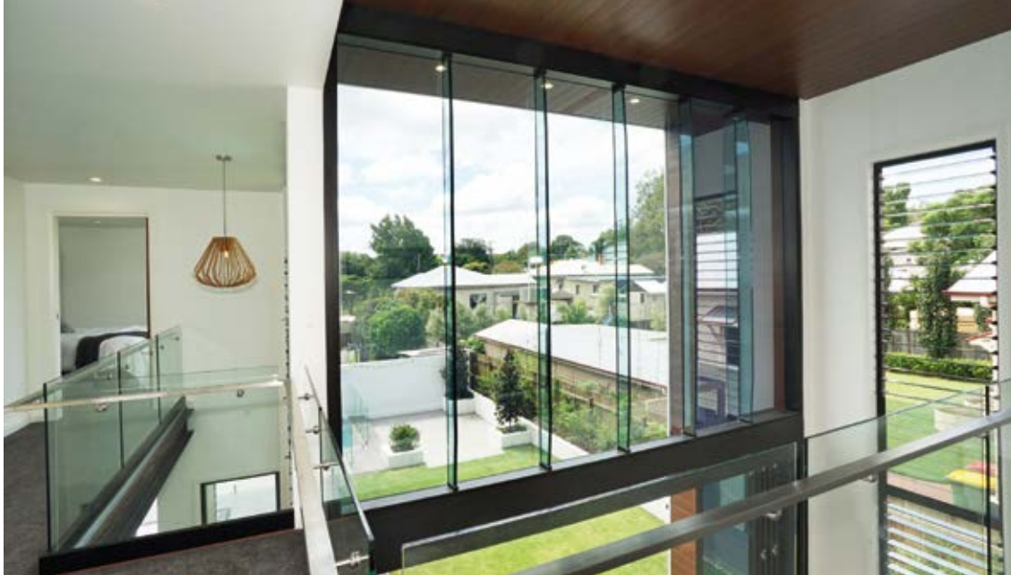
◀ Finned glazing & 050 Series Louvre Windows (Photo courtesy of Valdal Projects)
