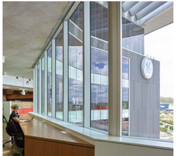
▲ Internal view GE Headquarters Springfield. GJ Solarplus (Low E on Grey) TwinGlaze units
